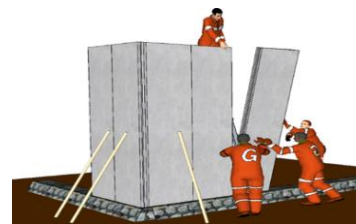
Figure 9. Panel Installation Method from Independent Modeling
