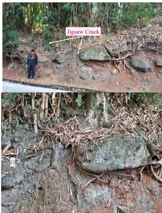
Figure 7. Observation Station ZI-2002 showing a debris avalanche deposit characterized by a jigsaw-crack structure.
